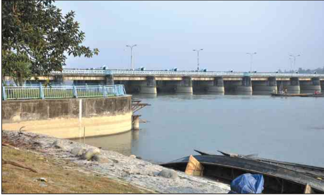
Down Stream view of Tista Barrage.
